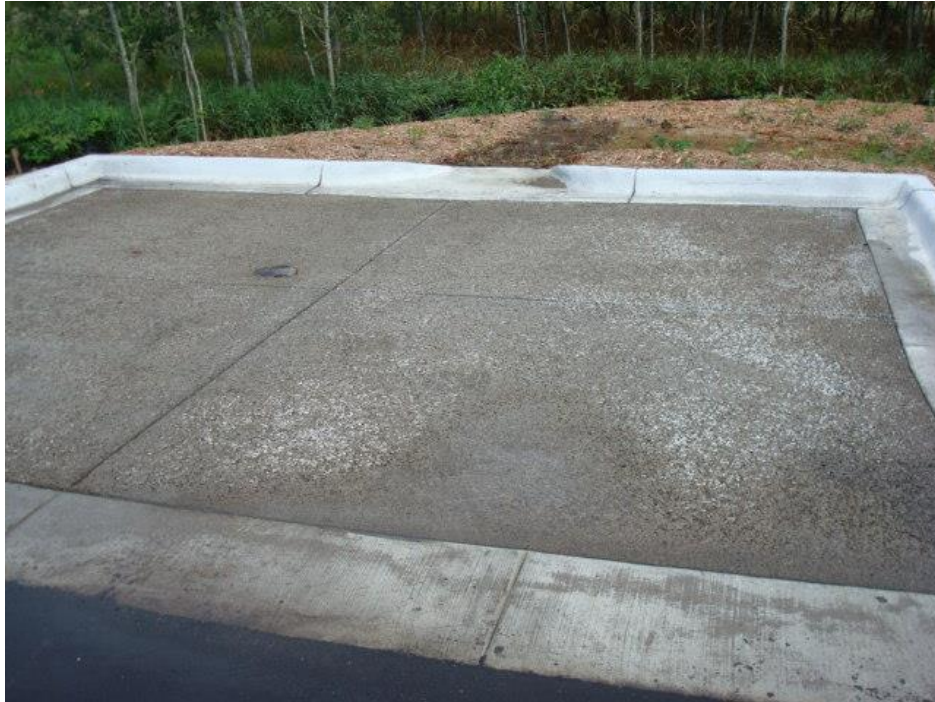
Blaine City Hall Pervious Concrete Fire Truck Turn Around
