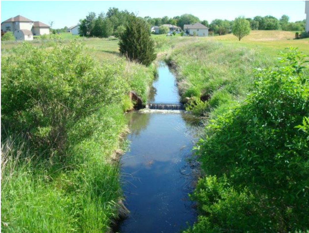
Structure on Ditch 58
