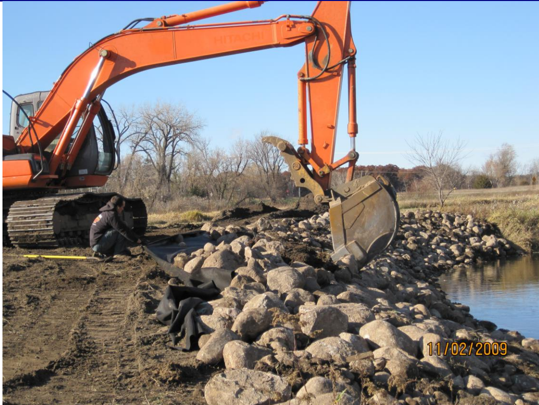
Crown Point bank stabilization fall 2009
