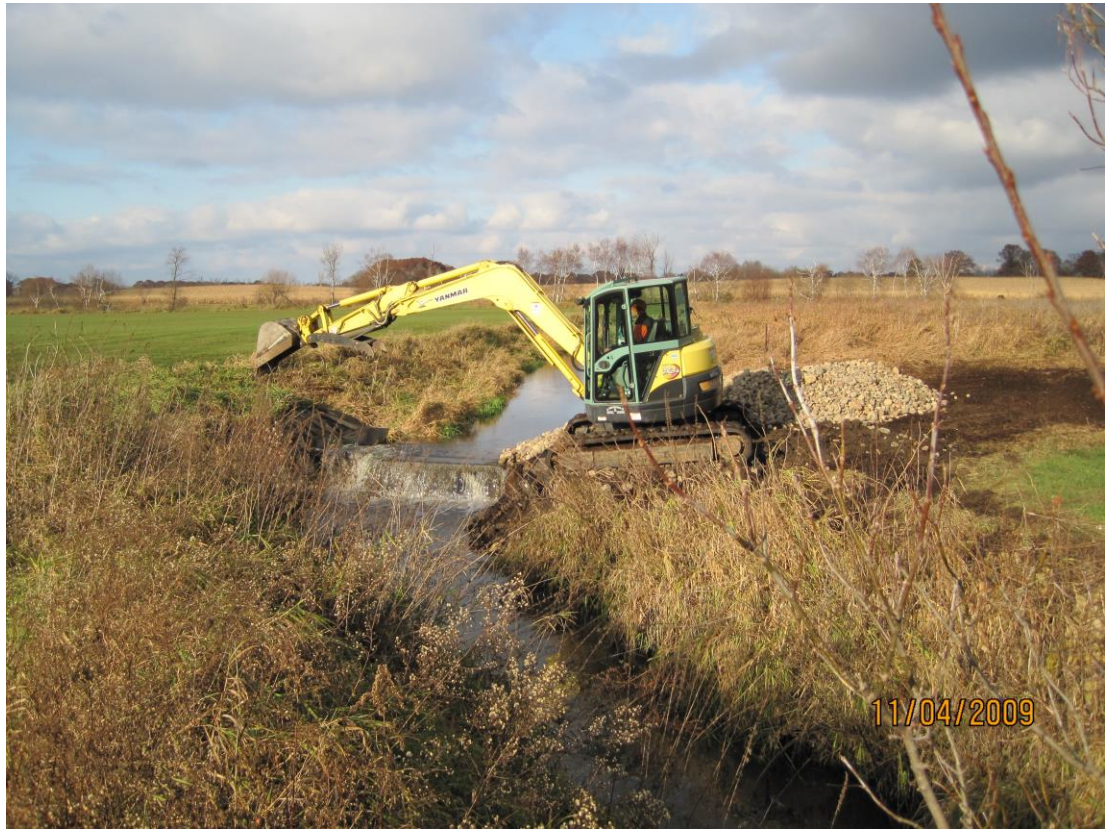
Timberline Structure Repair, 2009
