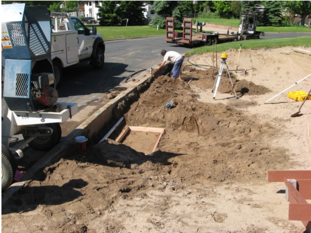
Crooked Lake Rain Garden Inlet protection box install , July 2010
