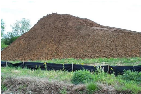
Silt fence around soil stockpile. Photo credit: Barry Tanning, Tetra Tech
