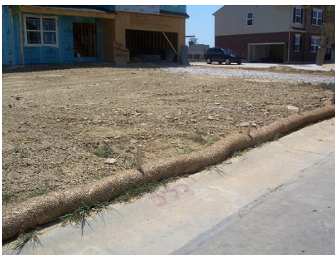
Make sure filter log stakes are spaced to prevent undercutting or bypasses. Leave stake tops extended along sections to prevent drive-overs. Photo credit: Barry Tanning, Tetra Tech
