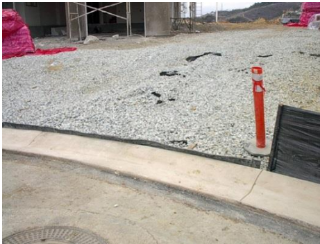
Good application of rock exit pad. Note short section of material against curb that is keeping rock from leaving site. Photo credit: John Kosco, Tetra Tech.
