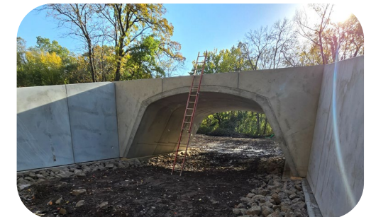
CRDRP Bridge Upgrade (Anoka Co Parks)
