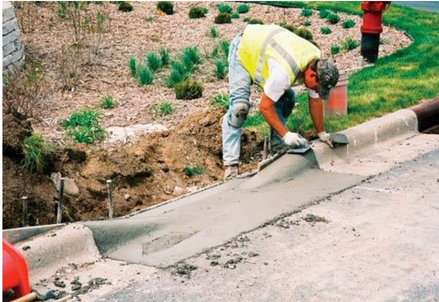
Cuts in the curb allow stormwater to enter the gardens from the street.
